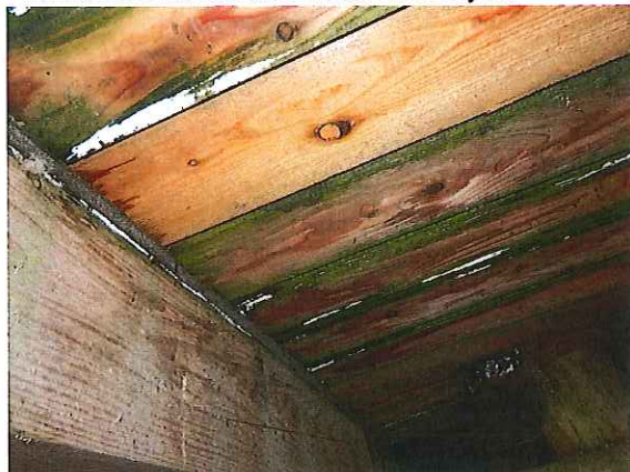
KLWI901_A_2019H_BELAG F-3 UNTEN LINKS PILZMYZEL
