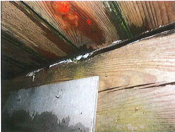
KLWI901_A_2019H_LT-3 F-4 HINTEN LINKS PILZMYZEL
