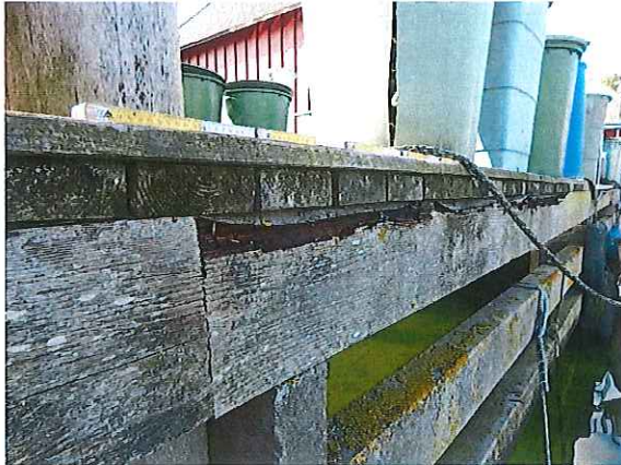
KLWI901_A_2019H_LT-1 F-4 LINKS OBERKANTE VERFAULT
