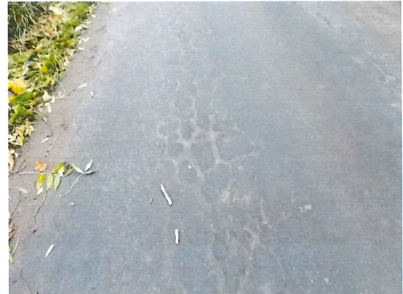
ZIER002_2015H_GERISSENER-ASPHALT
