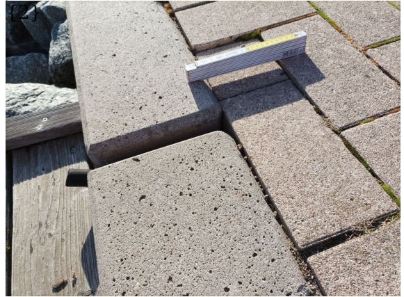
KLWI902_A_2023H1_ABSACKUNG-PFLASTER
